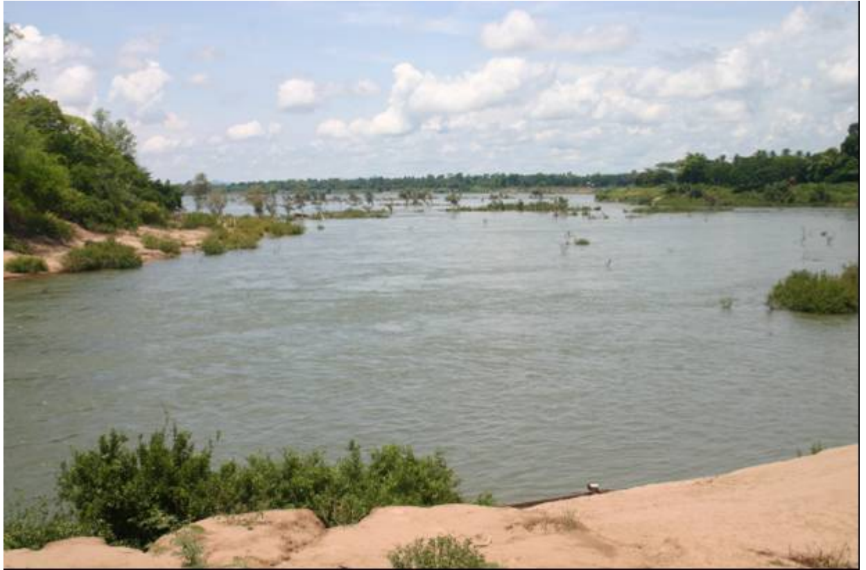
Dam site looking downstream
