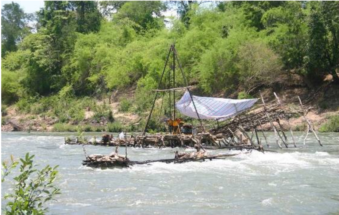
Hou Sahong – drilling rig for dam survey
