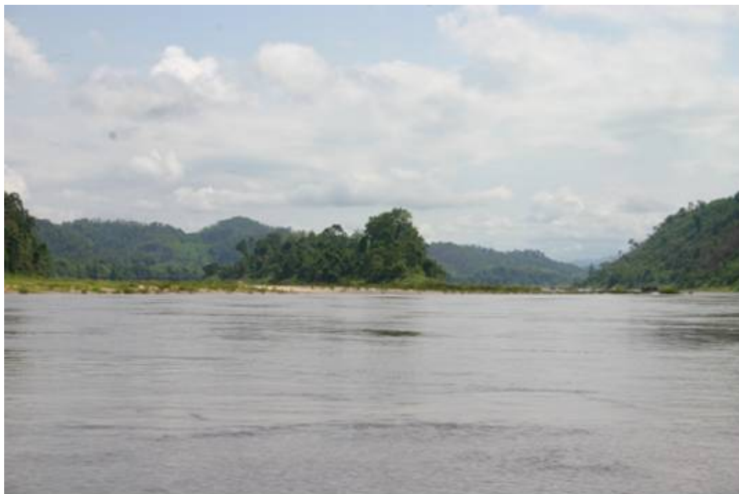
Pak Lay Dam Site Option 1 – looking upstream
